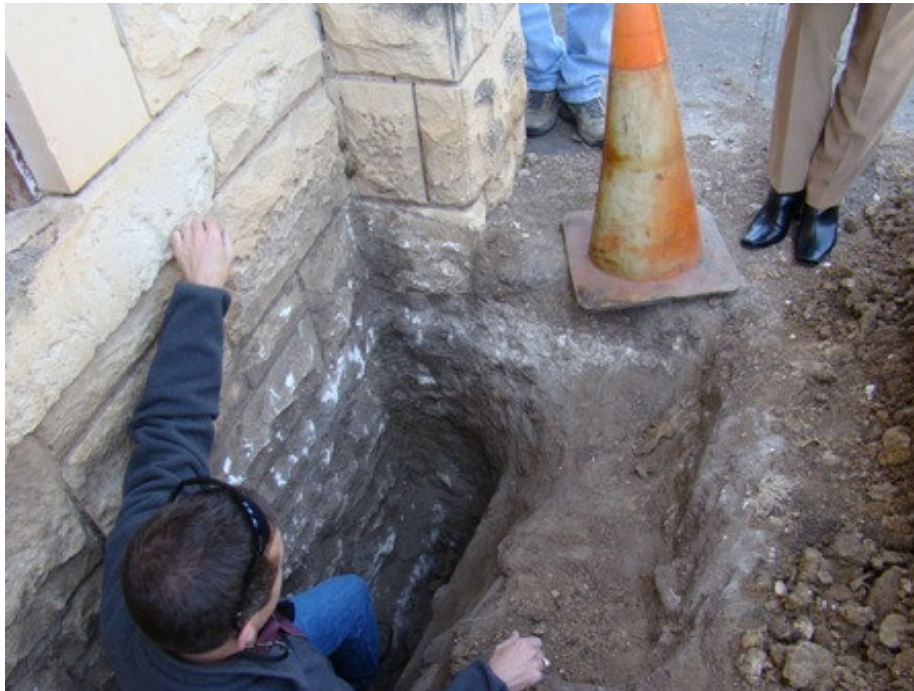
Foundation inspection pit.
