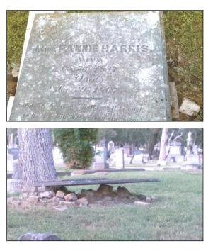
ground below grade. A concrete slab was poured and an inner wall of cinder block was erected to support the original bricks that form the outer wall. The ledger slab will soon be re-installed. All stages for the work were photo-documented. We all hope that these efforts will preserve Miss Harris's box tomb for the next 146 years.
