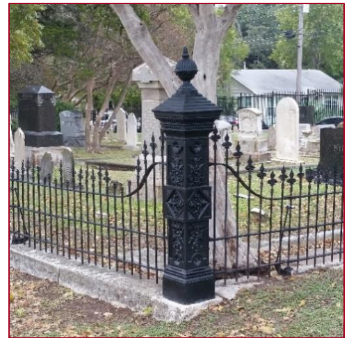
After damaged base has been repaired
