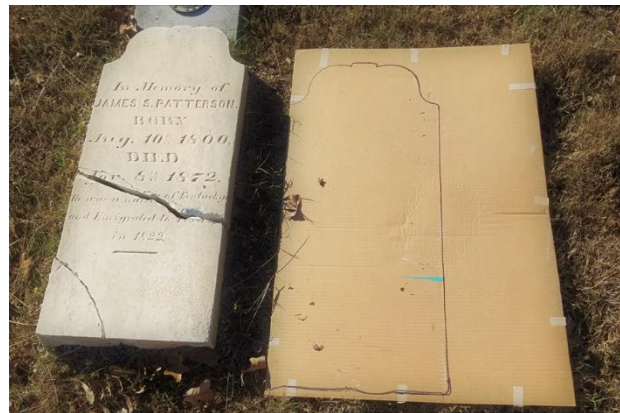
Top: Keith Crippen prepared a template of the Patterson gravestone for a cradle.
